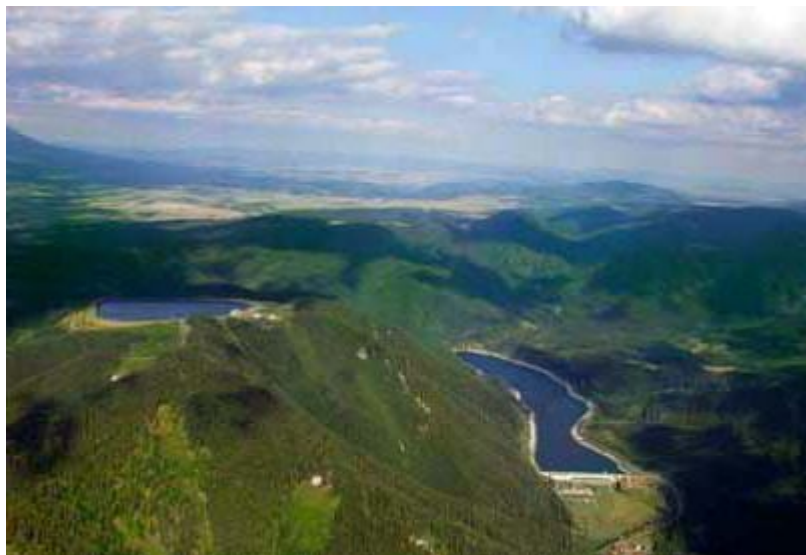
Figure 1 – Pumped storage hydro power plant (PSHPP) Čierny Váh [2]
